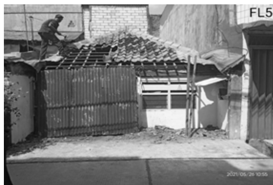
Figure 2. House Renovation: Photo submitted by Teenager 4
